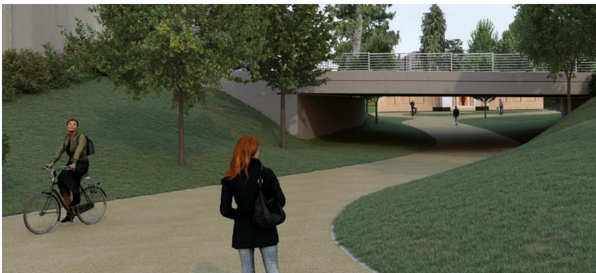
Image 4.8: Urban Realm Upgrade at North Circular Road Underpass
